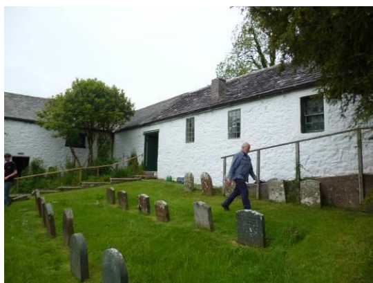
Fig.1: 1745 school room to right and 1731 stables to left, from the east
