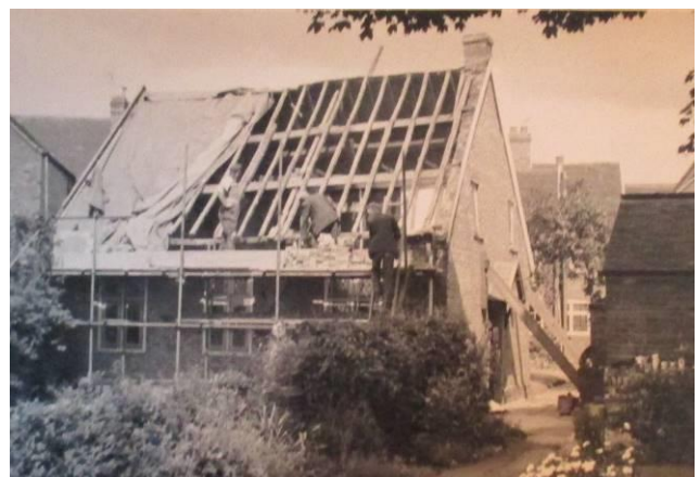
Figure 3: Roof being replaced, 1959.
