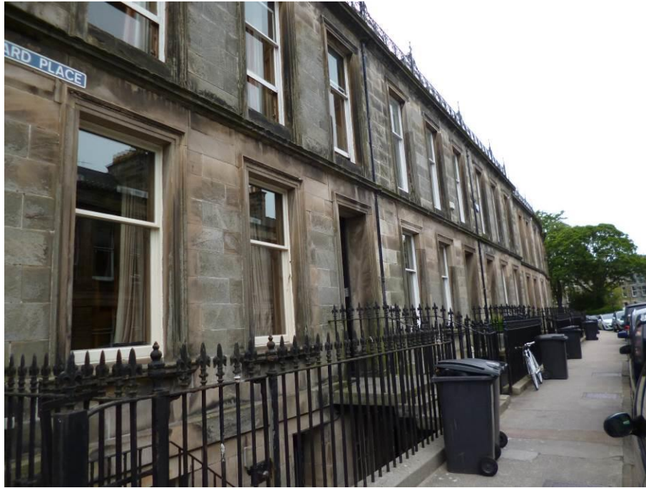
Fig.1: the meeting house is part of a formal terraced street
