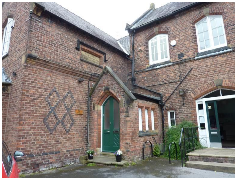
Figure 1. Detail showing the original entrance, brick diaper decoration and the stone plaque.
