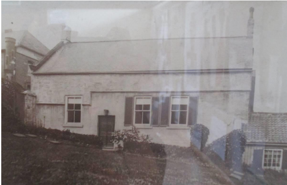
Figure 1: Meeting House rebuilt in 1844 (Pontefract MH Archive)
