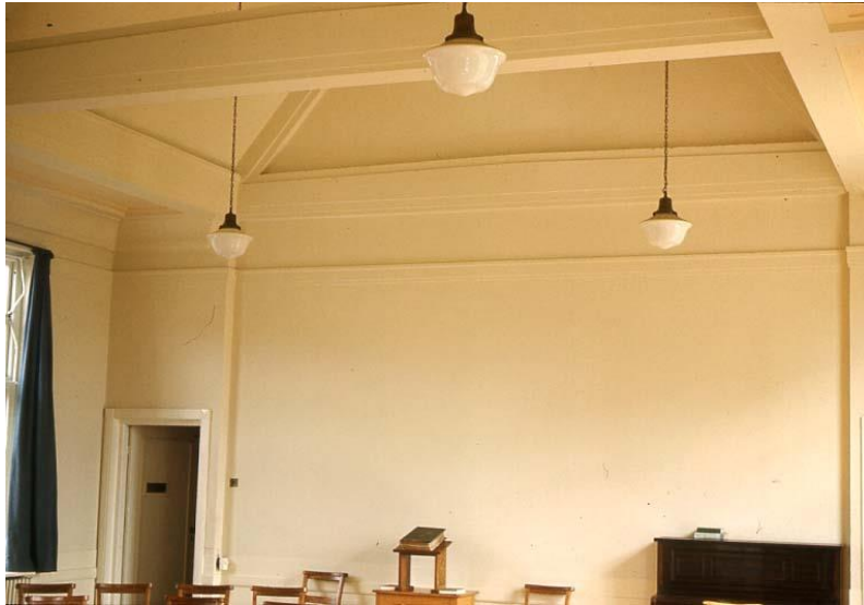
Figure 1: The interior of the meeting room prior to the installation of the suspended ceiling (Northfield MH Archive)
