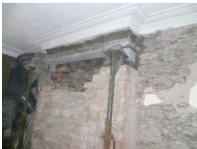
Figure 1: Removal of chimney breast c2000 (Leyburn MH Archive).
