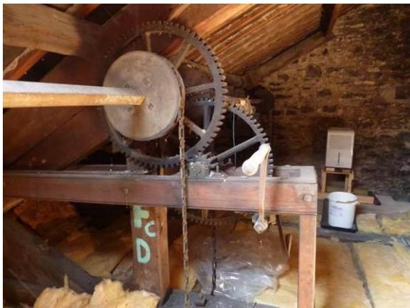
Fig.4: Lifting gear in the roof
