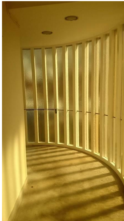
Figure 1: Access to the first floor via the oriel window. North is to the left.
