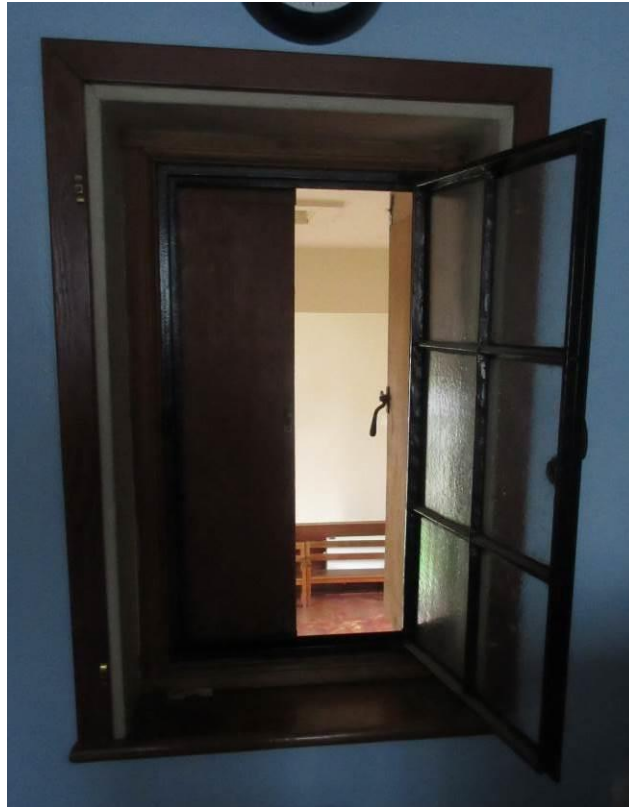
Figure 2: Window opening from upper classroom to meeting room
