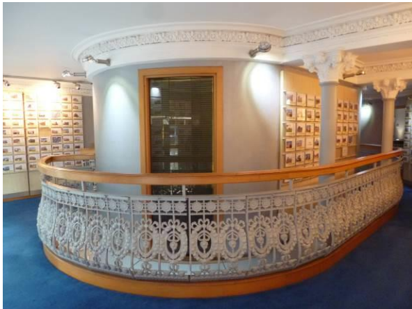
Fig.1: gallery balustrading re-set c.2000
