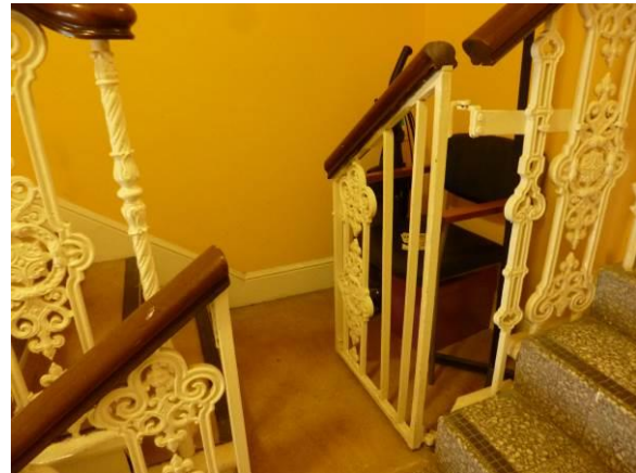
Fig.2: original gate in stairs to former gallery
