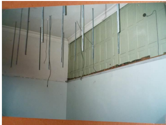
Fig.2: panelled shutters in situ above suspended ceiling, 2007 (Cockermouth Meeting House archive)
