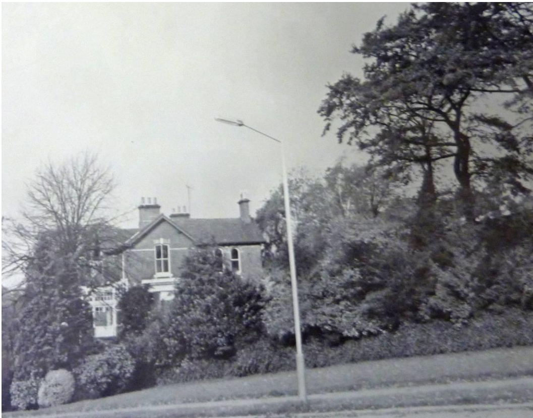
Figure 1 Goldwell Bank prior to demolition (Chesterfield meeting house archive)
