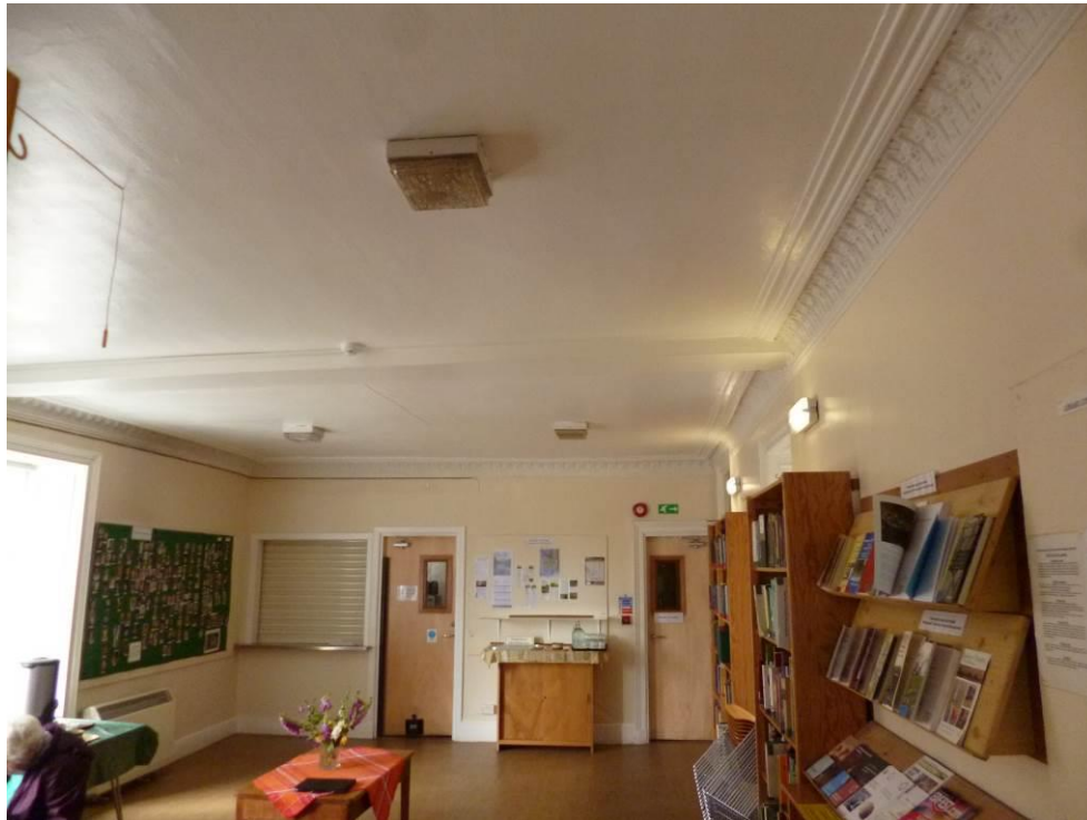
Fig.2: The library is in a former tenement, with plaster ceiling cornice
